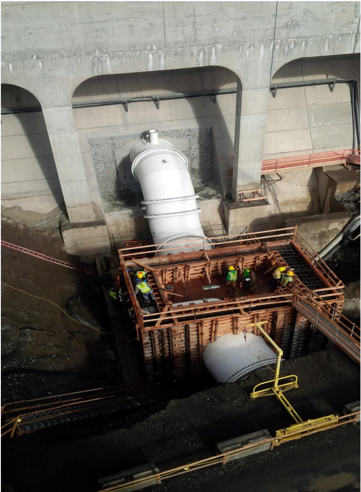
Forming room around 10' valve
