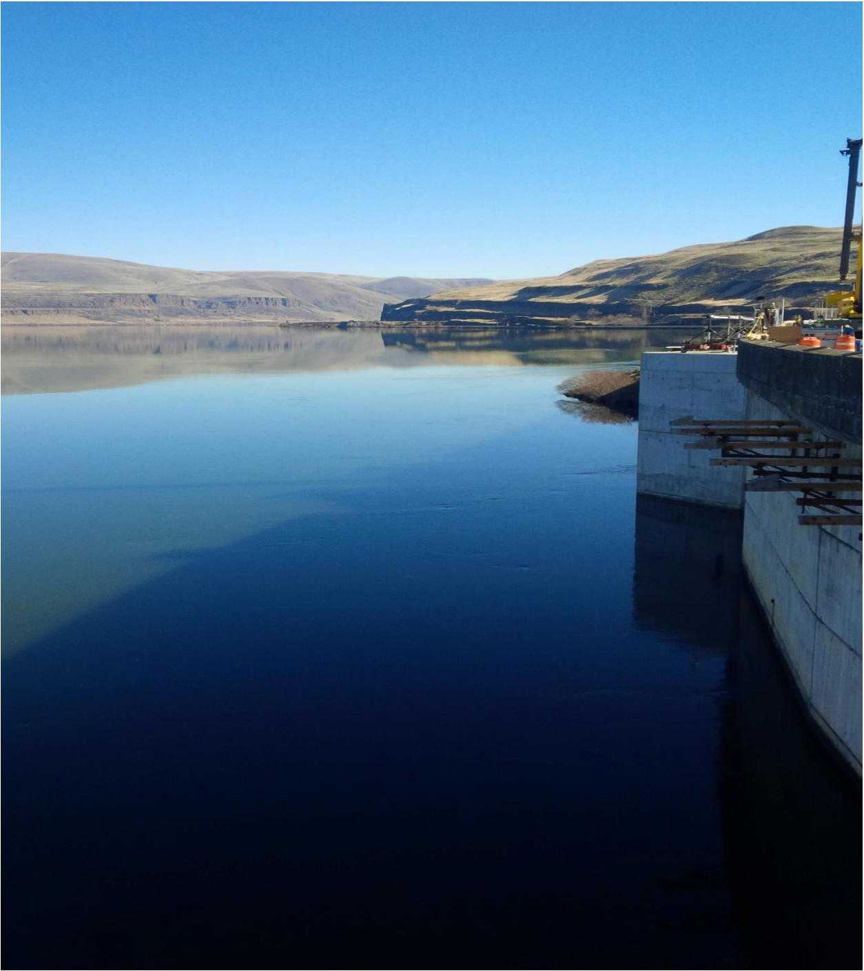
Finishing touches to AWS intake
